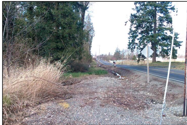
Photographs 14a and 14b. Roadside ditch that drains water from roadway and wetlands located adjacent to the Enumclaw Sportsman Park toward tributaries to Newaukum Creek within SMZ 1 (left – facing west from wetland; right – facing east from tributary).
