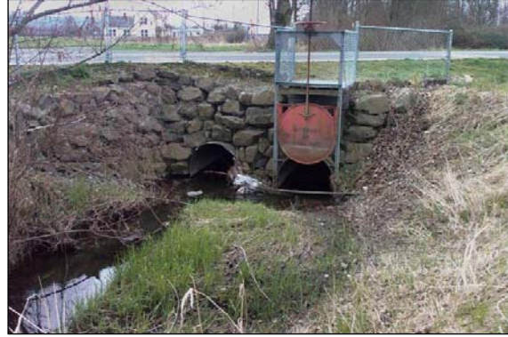
Photograph 8. Culvert under Warner Avenue connecting tributaries to Boise Creek in SMZ 3.
