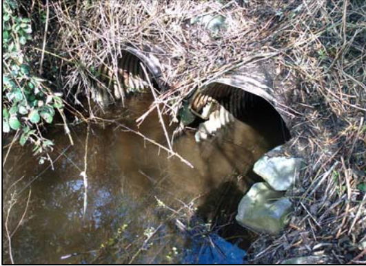
Photograph 16. Culvert under SE 440 th Street within SMZ 1.
