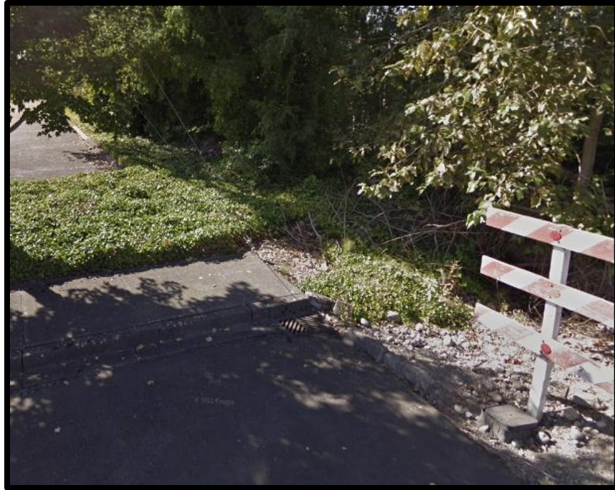
Element 1-2D: runoff is conveyed to the north alongside Watson St N (C), where it is then outlet into an unnamed stream. At this point the ¼ mile downstream limit is reached.
