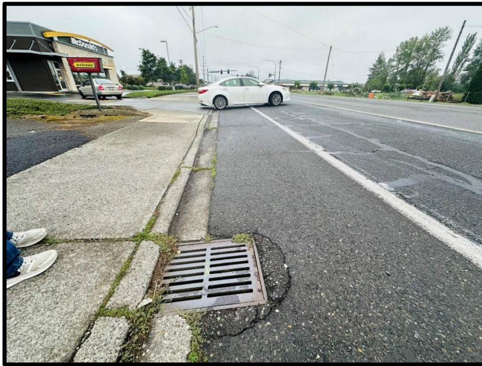
Element 1-2A: Stormwater reaches a catch basin on Roosevelt Ave E.
