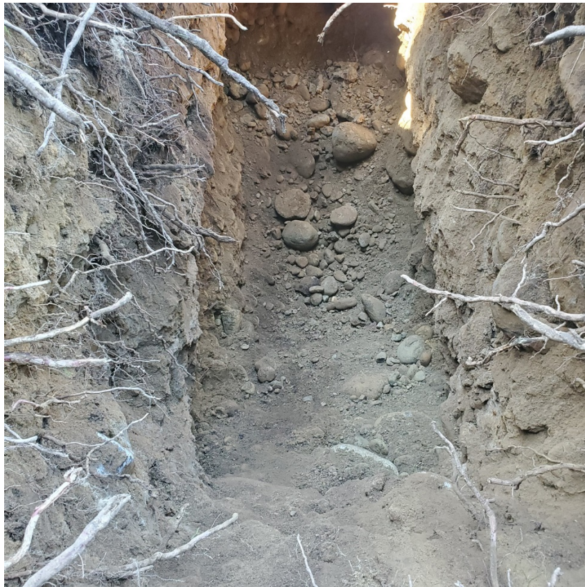
Image of soils encountered approximately 8 feet below the existing ground surface. TP-9 was terminated approximately 8 feet below grade. No groundwater seepage was observed during excavation.
