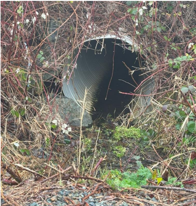
Figure 3-1: Downstream 48" Culvert, North Side of 440th Street
