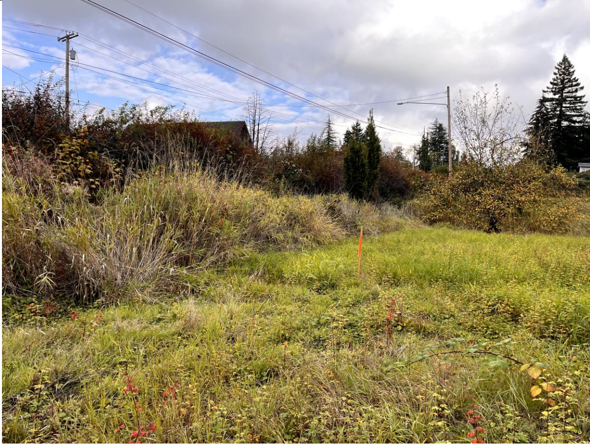
Filled/Failing Ditch Segment on Northern Portion of Subject Property (Note: Eroded Bank Indicative of failure, lack of channel to convey runoff away from site).
