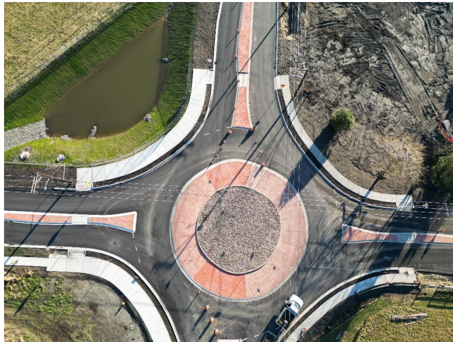
Figure 4- 244th Ave / Roosevelt Ave Roundabout Intersection Improvements
