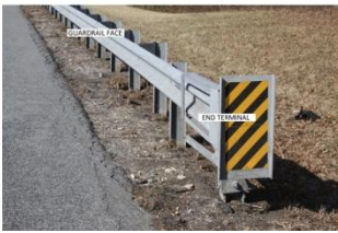
Figure 7- Guardrail countermeasure example Source: FHWA
