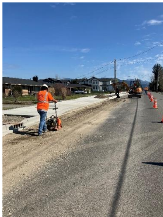
Figure 2-Sidewalk Fill Gaps Project Roosevelt Ave
