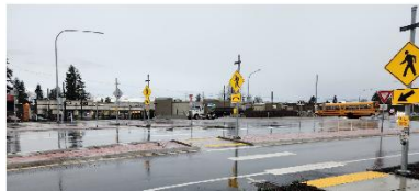
Figure 10-RRFB Examples Source: FHWA
