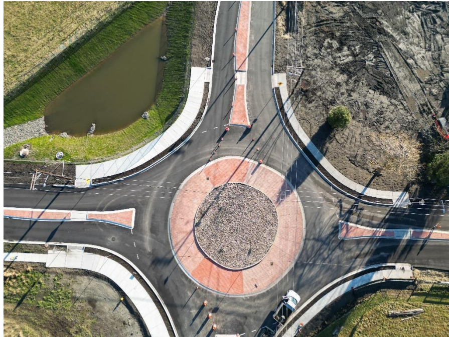
Figure 4- 244th Ave / Roosevelt Ave Roundabout Intersection Improvements
