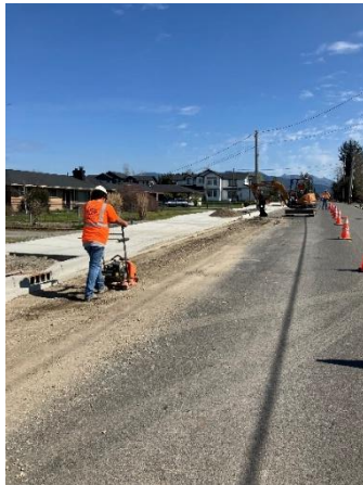
Figure 2-Sidewalk Fill Gaps Project Roosevelt Ave
