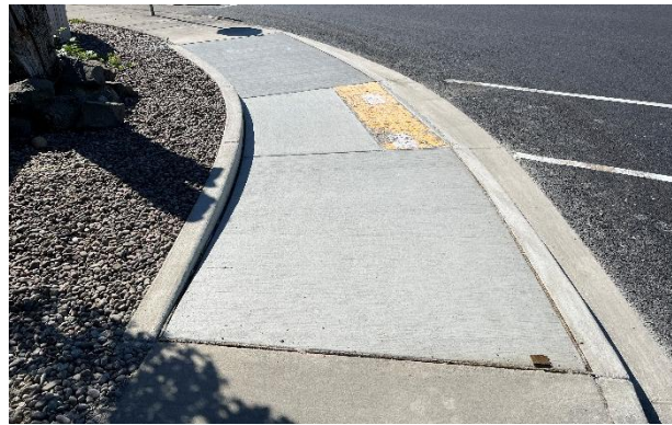
Figure 1-ADA Ramp Retrofit at Warner Ave and Blake St
