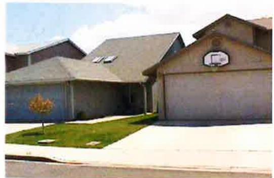
Garage dominates the front side leaving inadequate driveway length
