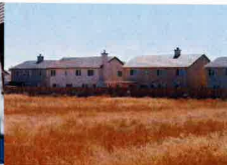
Figure 3B-6B: Don't do this This single family project does not have any variation in roof planes
